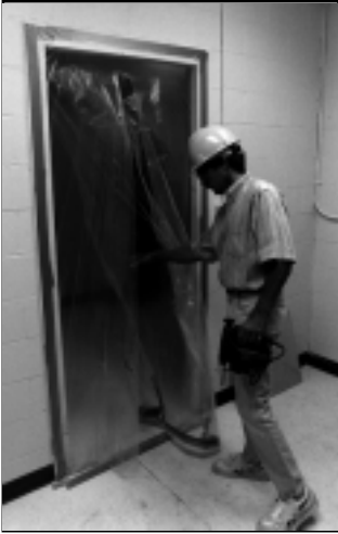
Close off entryways with an airlock.
